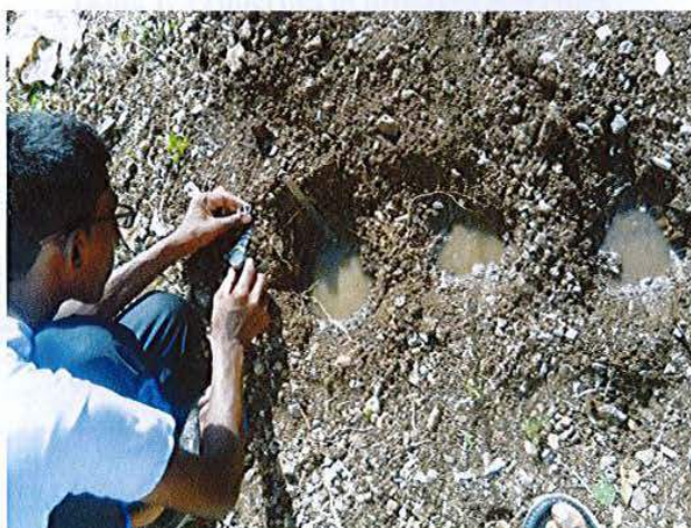
Figure 2.1: Step 3 of percolation test
