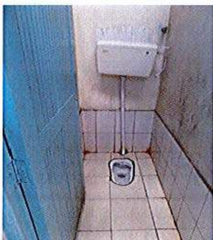
One of the public toilets constructed
